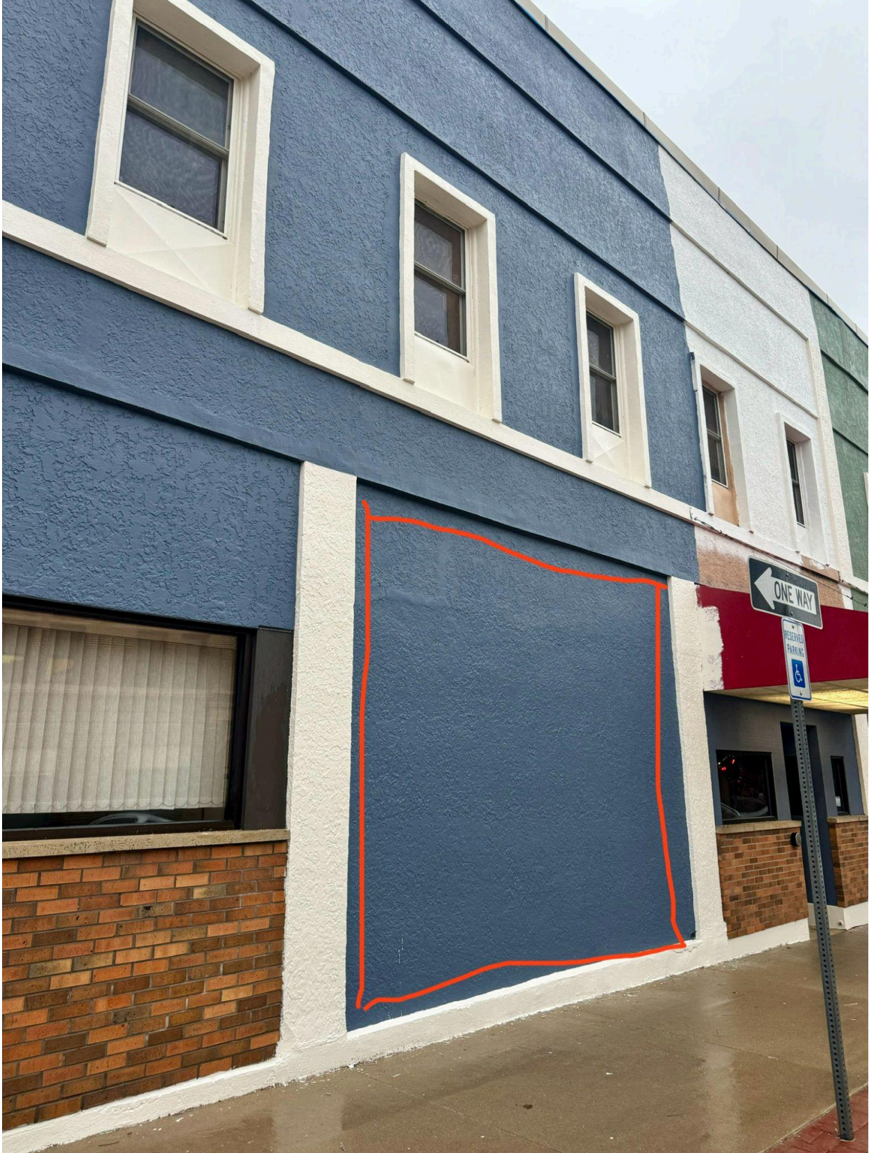
Current Site: (Side View)
