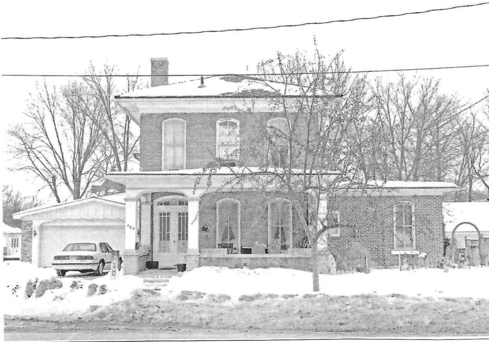
West Side (Mechanic Street View) Photographer Facing East
